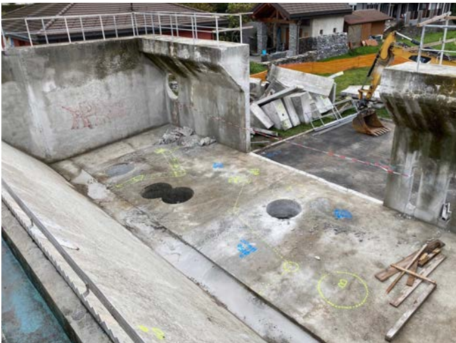
Above: The existing 1960s wastewater treatment plant, was modified and structures cut and reused. https://landezine.com/transforming-the-aproz-wastewater-treatment-system-into-a-playground-by-en-dehors/
