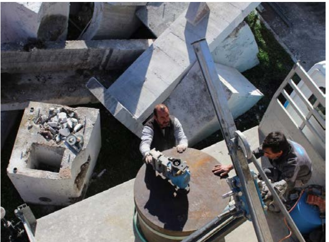
Above: The existing 1960s wastewater treatment plant, was modified and structures cut and reused. https://landezine.com/transforming-the-aproz-wastewater-treatment-system-into-a-playground-by-en-dehors/
