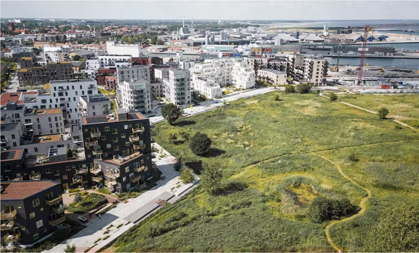
Above:View of the promenade and interface to the adjoining salt meadow. The promenade provides flood protection for the development. Source: https://www.archdaily.com/996753/the-south-harbor-of-koge-sla
